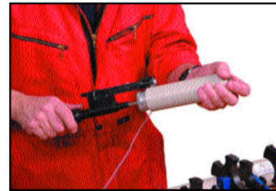
Using the peeling tool to chamfer the pipe
