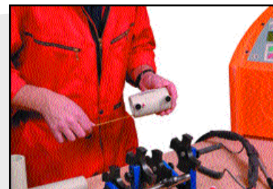
Measuring the fitting insertion depth
