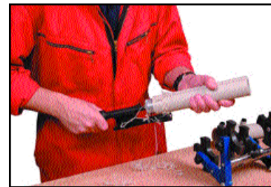
Peeling the pipe end prior to jointing
