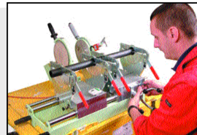
The heating element is removed and the pipes brought together
