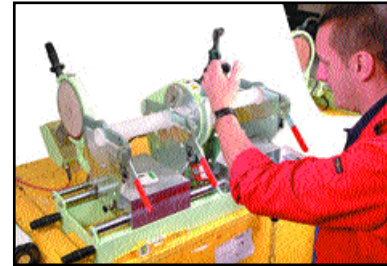
Planing the pipes
