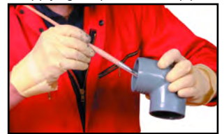
Brush applying cement to the fitting
