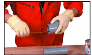
Measuring the insertion depth
