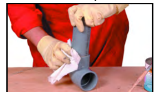
Wiping away excess cement
