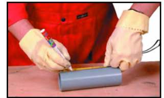
Marking the pipe end
