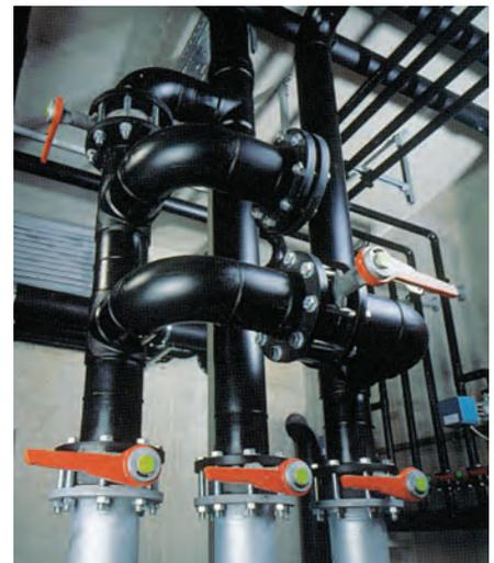
Polyethylene is no longer described by its density (LDPE, MDPE or HDPE), but by its resistance class according to ISO 9080 (PE 63, PE 80 or PE 100). Polyethylene piping systems are available from IPS in metric dimensions according to DIN 8077/8078 and DIN 16962.
