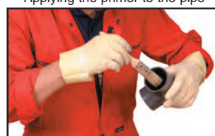
Brush applying cement to the fitting
