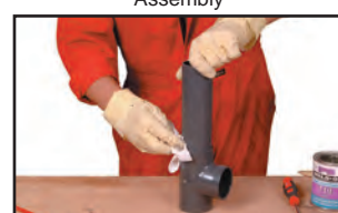
Wiping away excess cement
