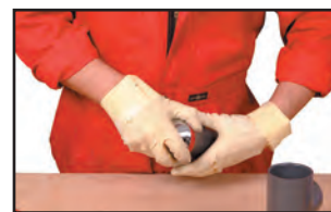
Chamfering the pipe
