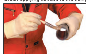
Brush applying cement to the pipe
