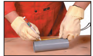
Marking the pipe end
