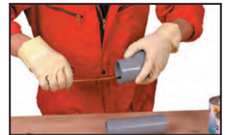
Measuring the insertion depth
