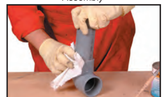
Wiping away excess cement
