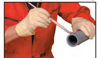
Brush applying cement to the pipe
