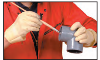
Brush applying cement to the fitting
