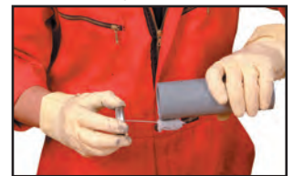
Applying the primer to the pipe
