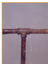
Leaking Joint
