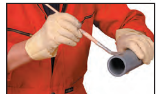
Brush applying cement to the pipe
