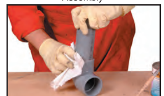
Wiping away excess cement
