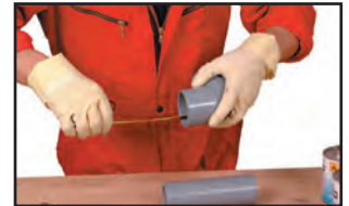
Measuring the insertion depth
