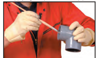
Brush applying cement to the fitting
