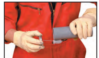
Applying the primer to the pipe
